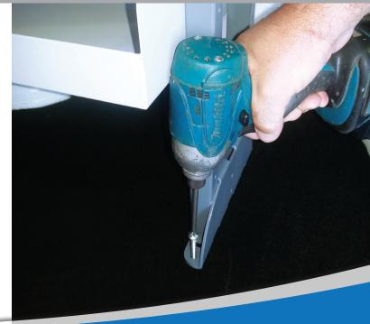
**Step 18:** Repeat step 17 for the remainder of the VAS Shelving System uprights. The VAS Shelving System is now securely attached to the vehicle floor.
