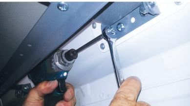
**Step 20:** Using a P3 Phillips head bit, secure the remaining shelves using Dog Head screws as shown in Step 15.
