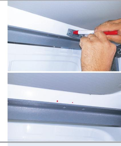
**Step 4:** Repeat this in three positions (preferably one at each end and one in the middle of the VAS Shelving System cross bar).
