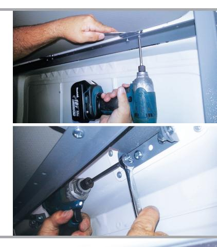
**Step 20:** Using a P3 Phillips head bit, secure the remaining shelves using Dog Head screws as shown in Step 15.
